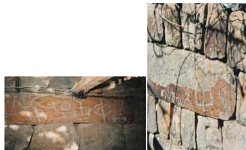
Fig. 4 Masterpieces used in construction
