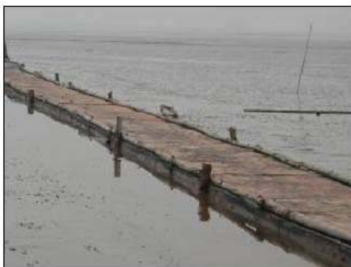
Fig. 3 Complete floating bridge
