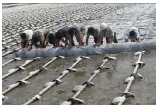
Fig. 7 Working photo of laying vacuum membrane
