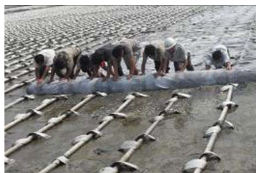
Fig. 7 Working photo of laying vacuum membrane
