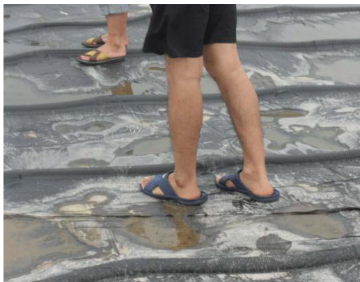
Fig. 10 Ground in half way of foundation treatment
