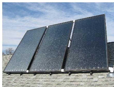
Fig. 1 Flat Plate Collector
