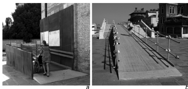
Fig. 4 Overlapping ramps: a. Ponte Paludo ; b. Temporary ramps for the Venice Marathon
