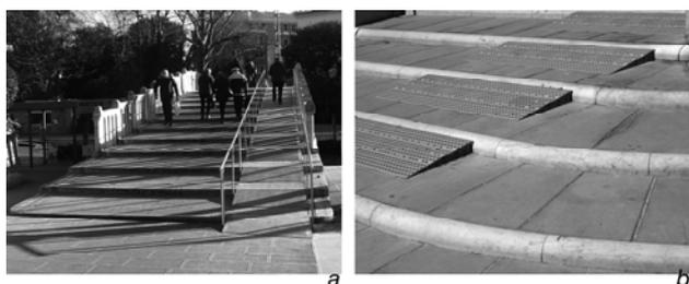
Fig. 3 Removable platforms: a. *Ponte Papadopoli*; b. *Ponte di San Pietro* with small plastic platforms
