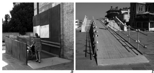
Fig. 4 Overlapping ramps: a. Ponte Paludo ; b. Temporary ramps for the Venice Marathon
