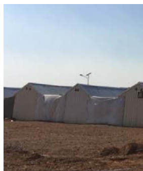
Fig. 22 Enclosed outdoor area [15]
