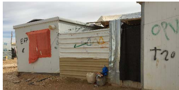
Fig. 7 A covered window to protect the privacy [13]
