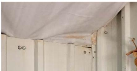
Fig. 14 Sharp edges in cladding [15]
