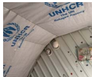
Fig. 17 Ventilation pipes closed [15]
