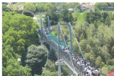
Fig. 12 Existing suspension pedestrian bridge
