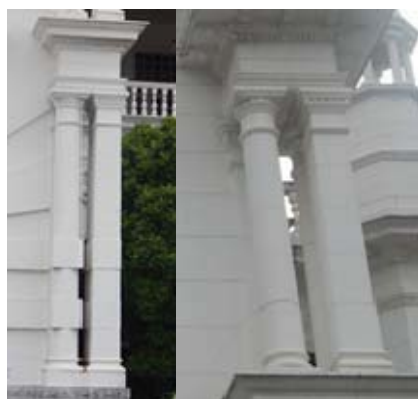
Fig. 10 The column capital of egg and darts molding
