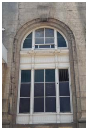
Fig. 24 Voussoir circular arch window with lion figurines, dentils and eggs and darts molding as detailing
