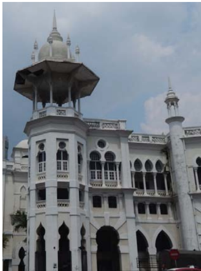
Fig. 17 Ground floor shows ogee arches, horseshoe arches and pointed horseshoe arches while the first floor shows double horseshoe arches and pointed horseshoe arches. At the roof top where there are dome chhattri which supported by multifoil arches
