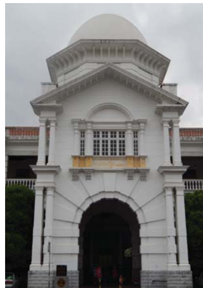
Fig. 20 Voussoir round arches in Ipoh Station
