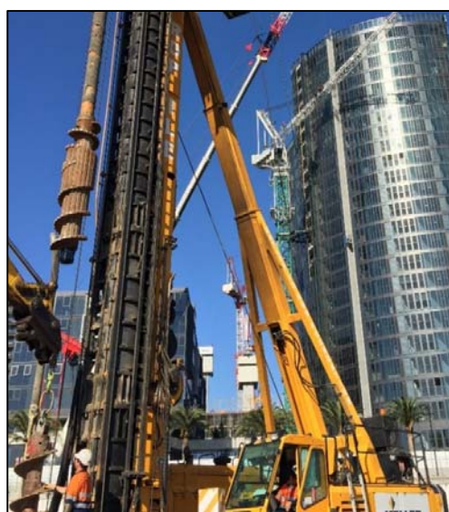
Fig. 7 Keller's modified DD drilling head
