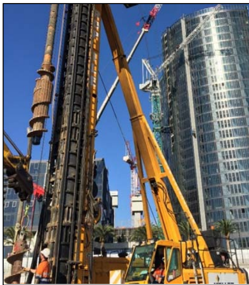
Fig. 7 Keller's modified DD drilling head
