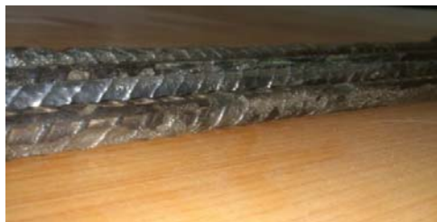
Fig. 4 Cleaned rebars after corrosion
