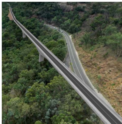
Fig. 7 Completed bridge in relation to existing road
