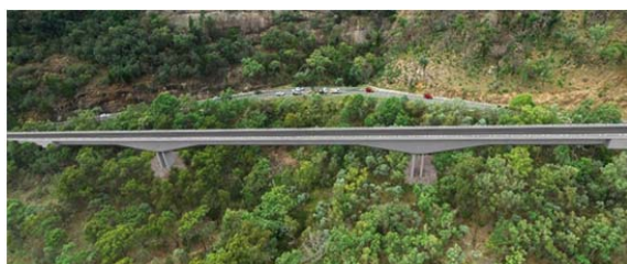
Fig. 1 (b) 3D view of the completed bridge from bottom of slope
