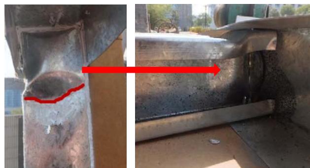
(a) Distortional buckling of W-1 CFS
