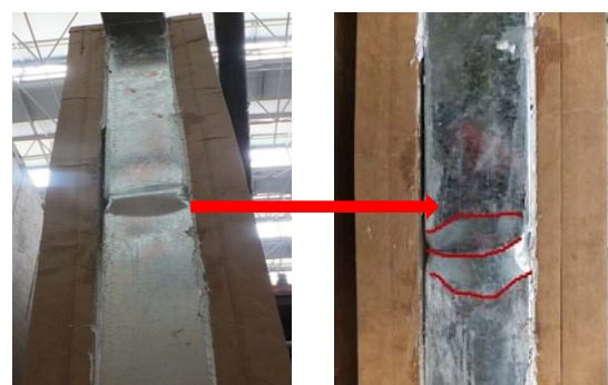
(b) Local buckling of W-2 CFS
