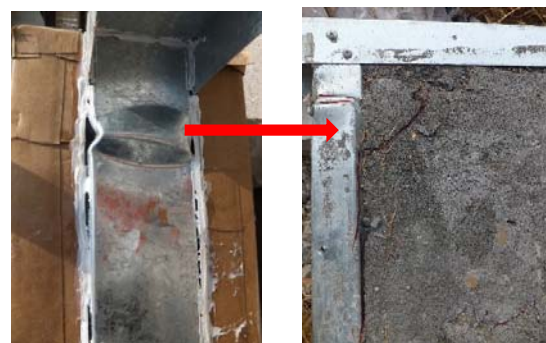
(c) Local buckling of W-3 CFS
