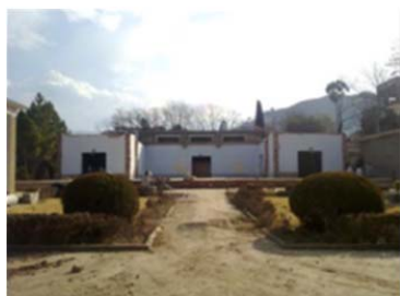
Fig. 9 Ongoing re-building and rehabilitation of Swat Museum by the Italian work [8]
