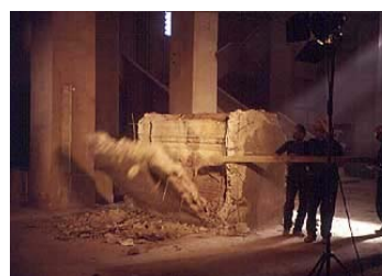
Fig. 5 Beirut National Museum. Rehabilitation after the civil war (1975-1991). Removing the cement box which covers a Roman Sarcophagus [4]
