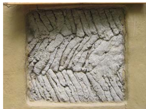
Fig. 10 Adobe and stones were provided walls
