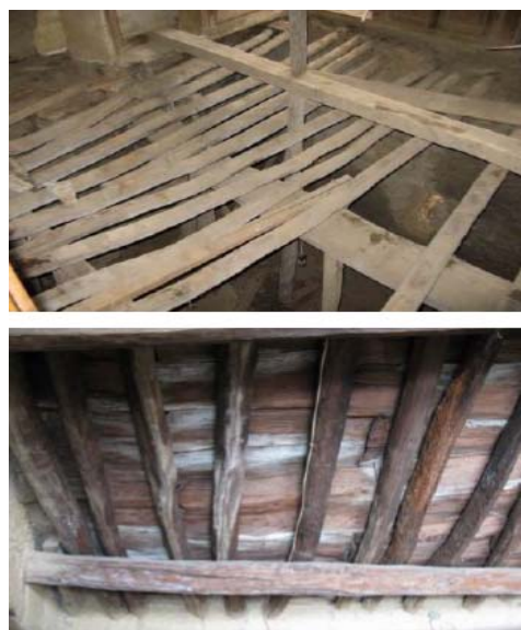
Fig. 11 The structure of roof at first until the end
