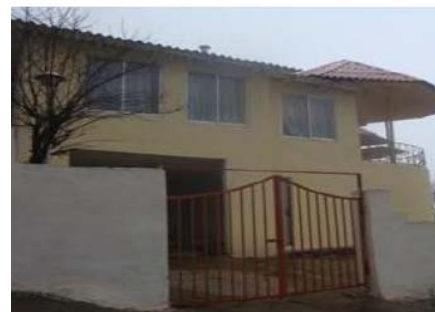
Fig. 14 New construction in staircase structure of Masouleh
