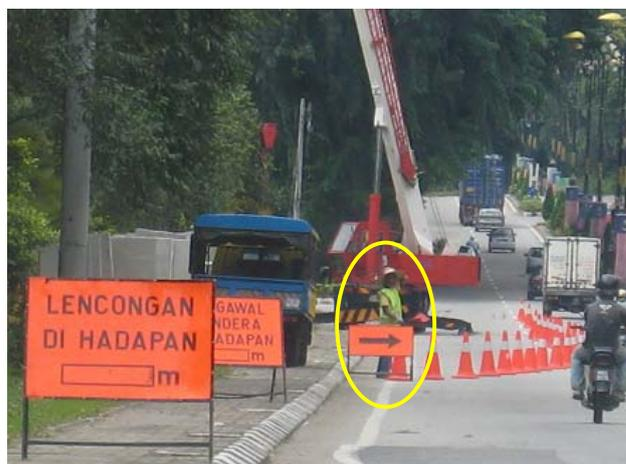
Fig. 1 Flagman is positioned in the work zone
