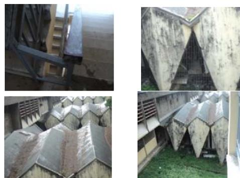
Fig. 1 Corrosion attacks of steel and concrete structures in the University of Lagos, Nigeria
