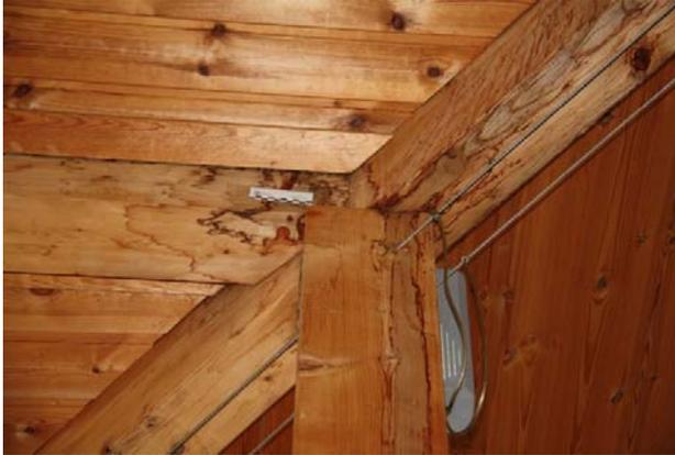
Fig. 1 Convective moisture ingress through a leakage at the connection point of bay and timber frame
