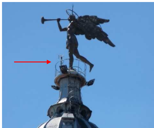
Fig. 3 View of the weather vane on the top of the bell tower of Lendinara; the red arrow evidences the location of the anemometer
