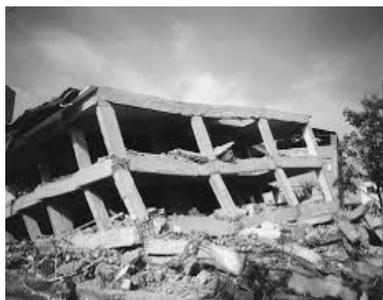
Fig. 5 Beam column Joint failure
