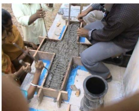
Fig. 9 Casting of beam column joint
